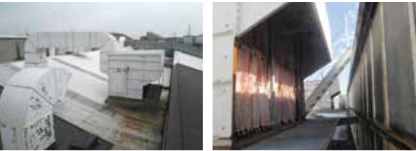
Painting booth exhaust duct High-performance filters Countermeasures against paint mist from the painting process
