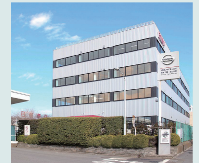
Tsunami evacuation site -Head office building-
