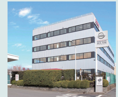
Tsunami evacuation site -Head office building-
