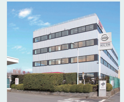
Tsunami evacuation site -Head office building-
