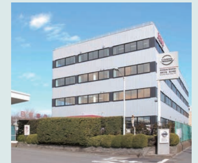
Tsunami evacuation site -Head office building-
